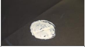
Roughen the area that the patch will cover with sandpaper. Spread a thin layer of adhesive over the area and apply the patch.
